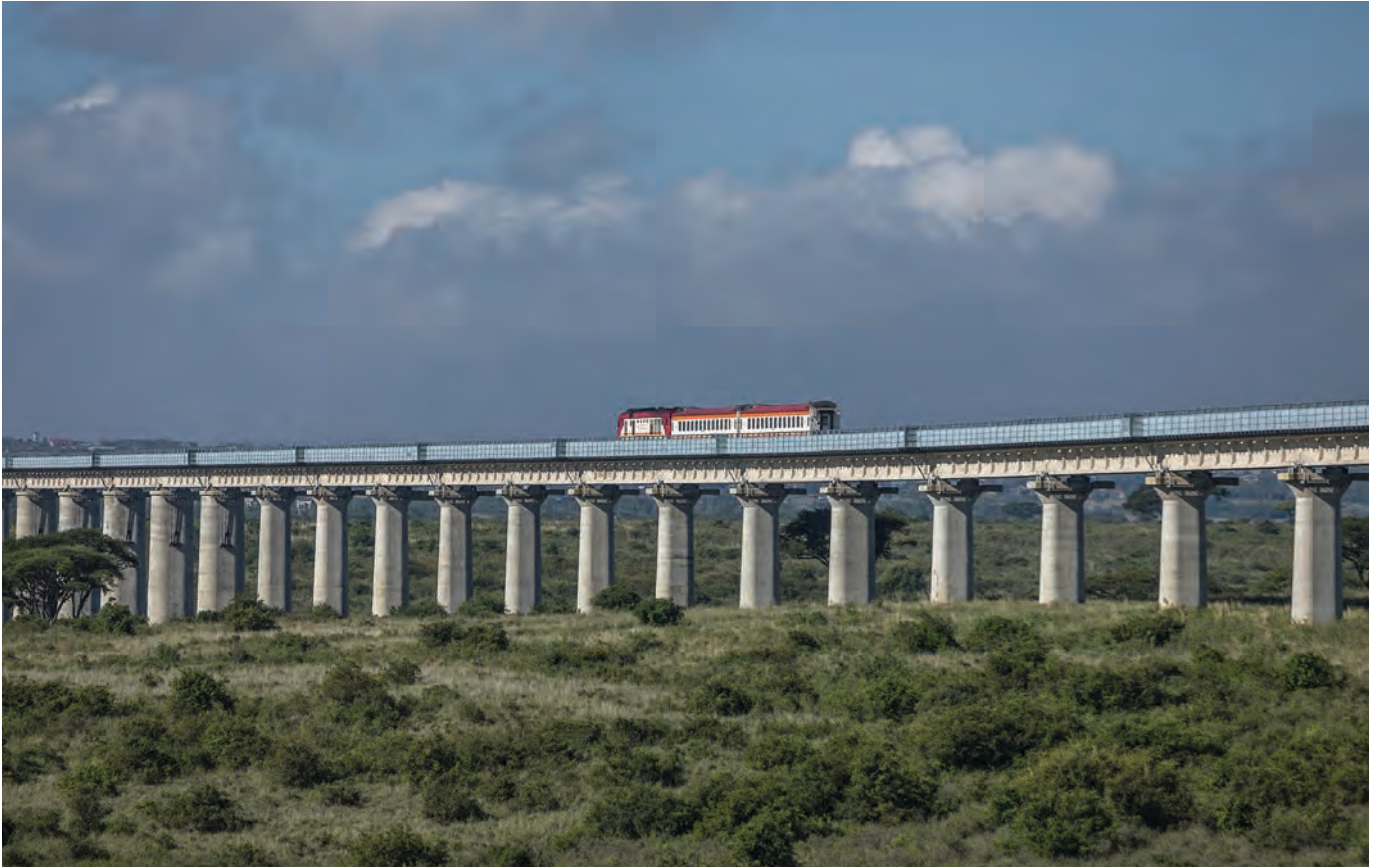
A train travels along the Standard Gauge Railway, funded and built by China, inside Kenya's Nairobi National Park on December 24, 2021. The railway is one of several major infrastructure development projects China has financed in Africa in recent decades. (Photo by Brian Otieno/New York Times)
