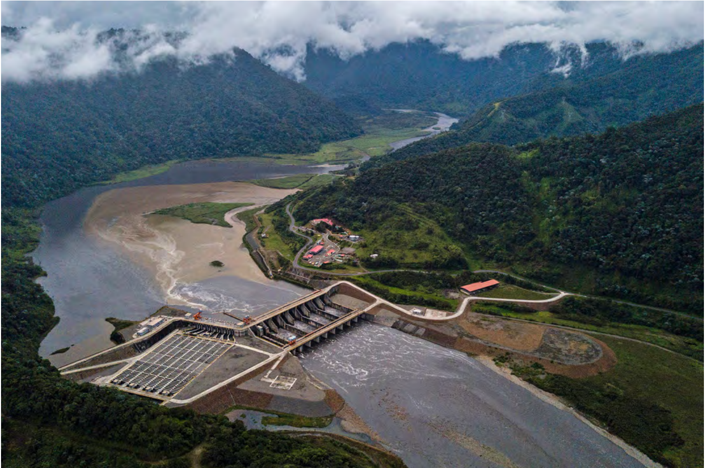
The Chinese-constructed Coca Codo Sinclair hydroelectric dam project near Reventador, Ecuador, on November 25, 2018. The dam has never operated at maximum capacity and supplies less than 30 percent of Ecuador’s total annual electricity needs. (Photo by Federico Rios Escobar/New York Times)
